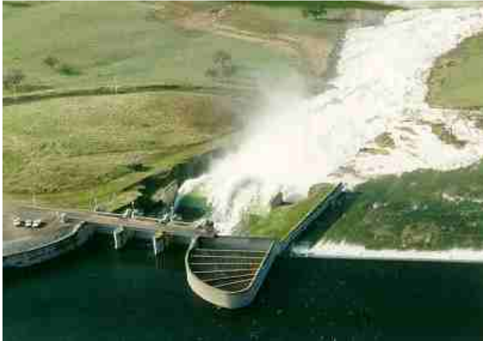
Figure 7. Tuolumne River cascading down spillway of New Don Pedro Dam in January 1997. Photo from CDWR.
