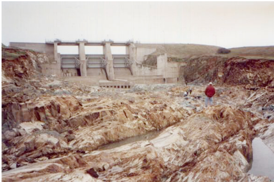
Figure 8. Channel scour effects downstream of Don Pedro Dam in March of 1997. Fish habitat improvement projects downstream of this site were obliterated.
